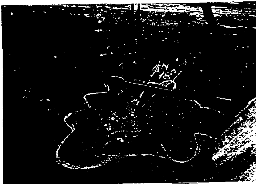
Picture 2. A photo of the effects caused by particles on the asphalt surface
